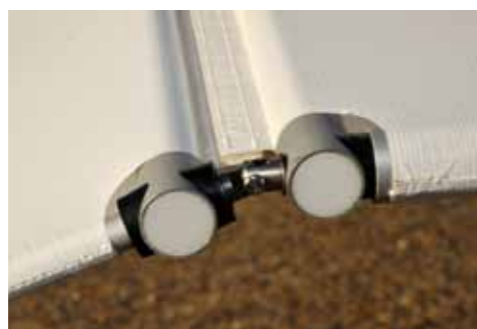
The Xlam fabric covering also serves neatly as an elevator gap seal. Note the plugged tube ends
